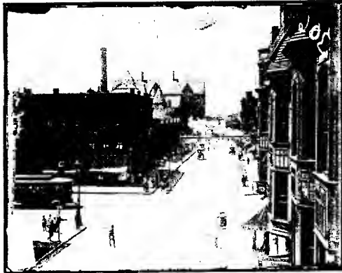
Figure 1. Looking west down 33rd Street (1909). Main Building is visible in the background to the left.
